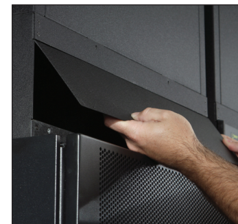
Removable blanking panels capture heat.
